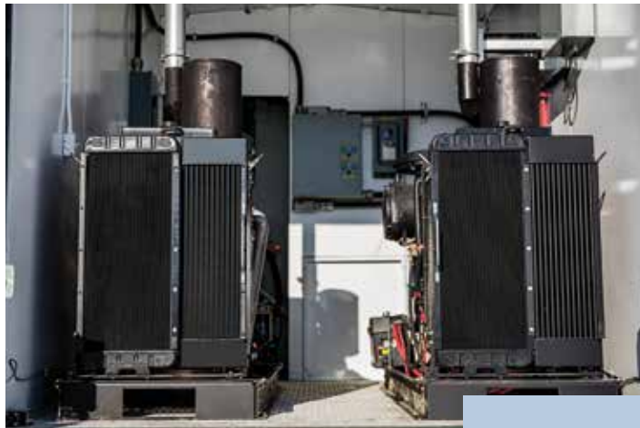
Frontier Power Products supplies the gen-sets as complete skid-mounted power units, ready for installation.
