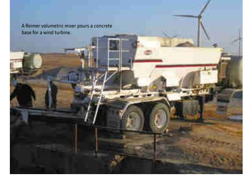
Reimer Mobile Mixers produce up to 57 cubic meters (75 cu. yds.) of concrete per hour and are designed and built to run continuously. "When you're mixing concrete at higher volumes at lower slump, at high production rates, you need an engine that can hold up to that kind of load and pressure," explains Steven. "We are happy with the torque curve of the John Deere engines, because they hold the load right where you need it.
